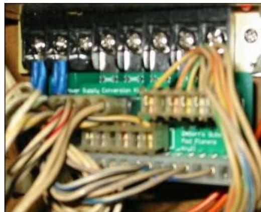
**Step Four: Hooking up 120 V.A.C. power to the new power supply...**
